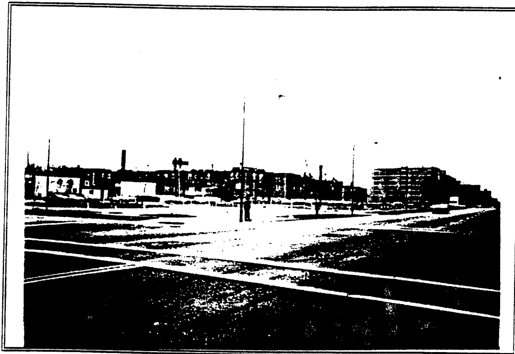
SUBJECT SITE SHOWING THE NORTHWEST CORNER
